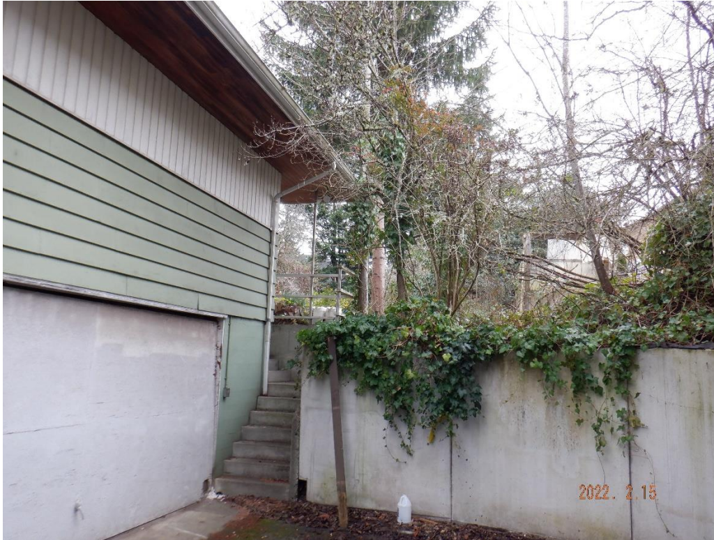
Trees #890 and #891 close to existing house
